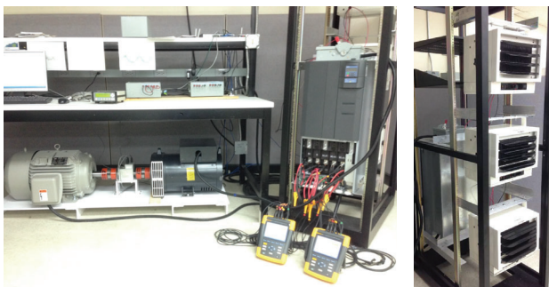
Image of entire system as well as connected heaters used as load bank
