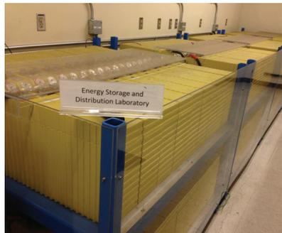
The load control hardware installed in the 1084 building is shown on the left. The 500kWh stationary battery energy storage system installed in the 1200 building is shown on the right.
