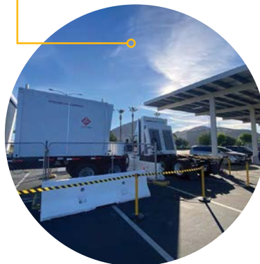
Refueling a Fuel Cell Vehicle at the CE-CERT hydrogen refueling station (rated to 700 bar, 500 kg of fuel)
