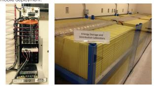
The load control hardware installed in the 1084 building is shown on the left. The 500kWh stationary battery energy storage system installed in the 1200 building is shown on the right.
