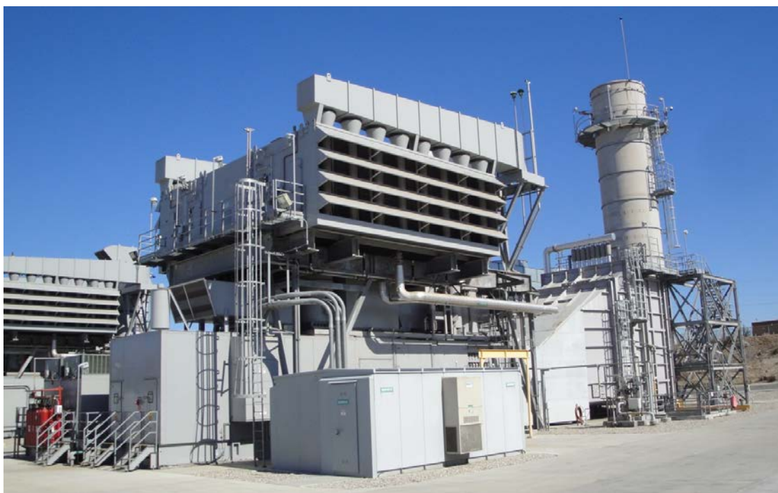
Figure 2-5: A 50 MW, Peaker Power Plant Using GE's LM6000 Turbine with SCR
